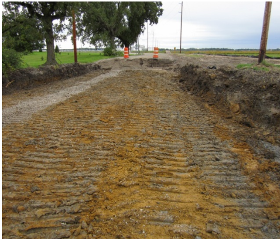
Image 1 – Subgrade Preparation
