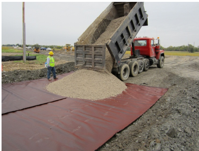
Image 3 – End dumping aggregate
