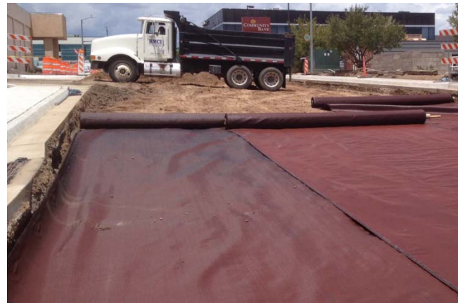
Image 7–Extending the Geosynthetic Reinforcement up a Vertical Face
