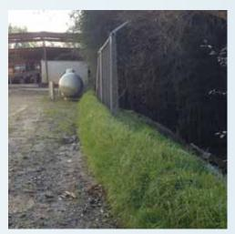
If vegetated, EnviroSoxx can be left in place as a permanent feature of the landscape. For temporary uses the FilterMedia can be incorporated into the soil, spread over the landscape, or returned to an approved composting facility.
