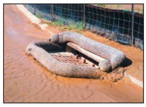
Curb Inlet Protection - Fine Silts Filtration
