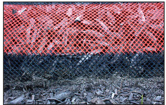
Close Up of Sediment Control
