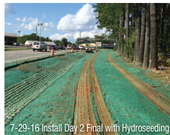
7-28-16 Install of Flexamat
