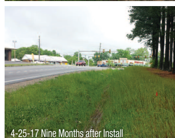
4-25-17 Nine Months after Install
