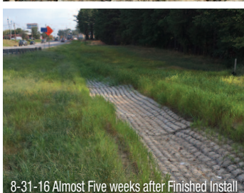
8-31-16 Almost Five weeks after Finished Install
