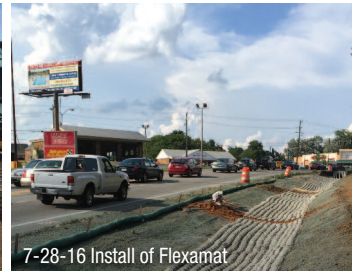
7-28-16 Before Install Laying Filtrexx
