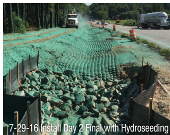
7-28-16 Install of Flexamat
